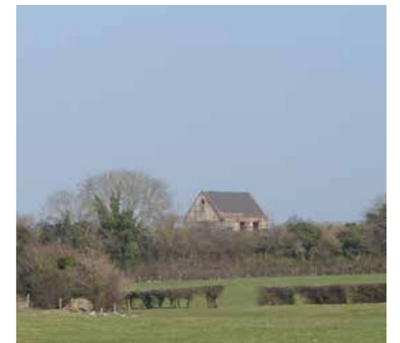
RPS 0700 Former School house, visible over the planted edges of the railway and the Royal Canal
