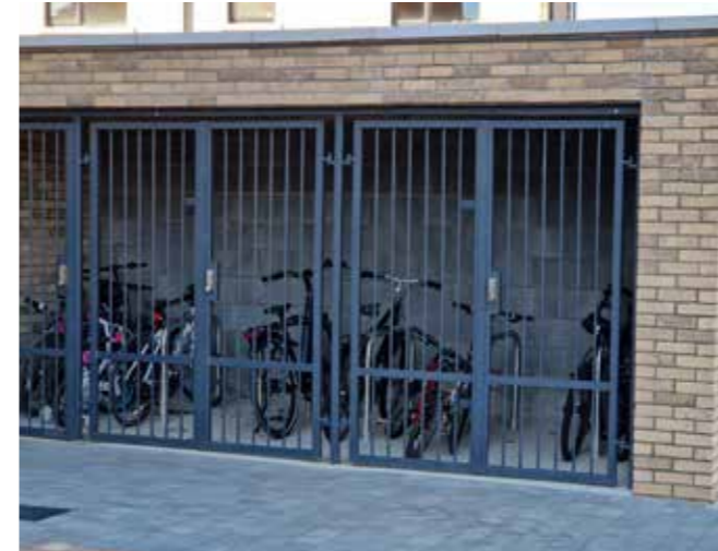
On street, gated bicycle stores with Sheffield Stands, for terraced houses are proposed within the streetscapes. Castlethorn have built similar bicycle stores in other projects, such as in Woodbrook Phase 1, located in Dun Laoghaire Rathdown County Council. The above precedent photo is from Woodbrook Phase 1.
